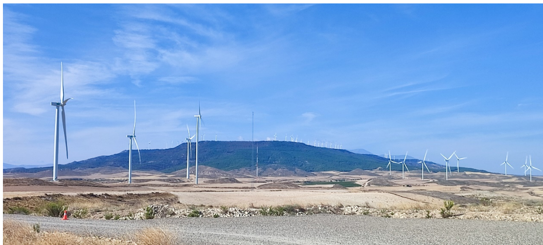
Figure 2: The El Campo wind farm
